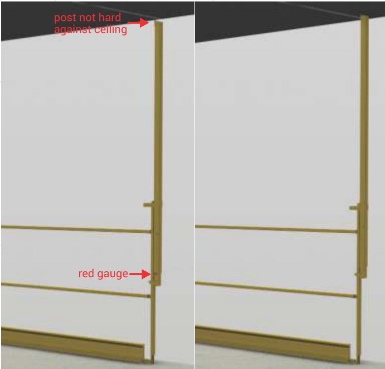
Incorrectly installed.
